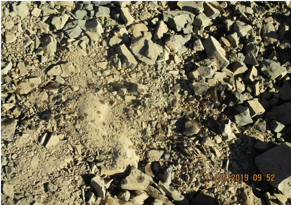
Photo: Minor oil spill at Section B of 132kV terrace.
