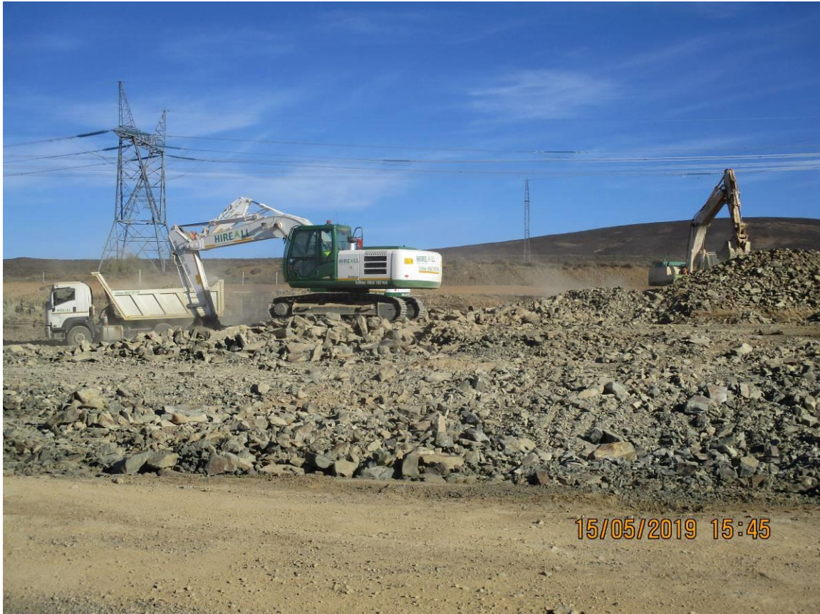
Photo: Bulk earthworks at Section B of 132kV terrace.
