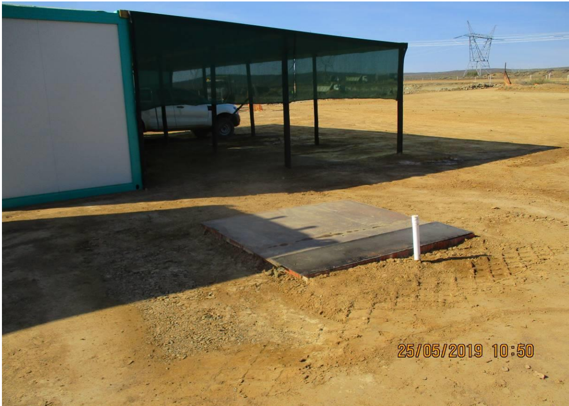
Photo: Constructed bund for underground septic tank.
