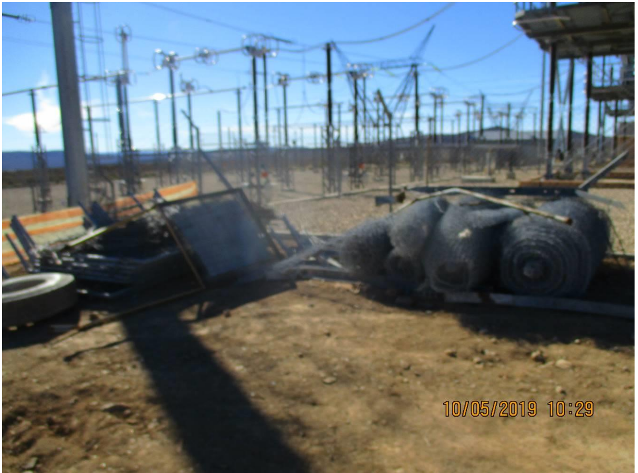
Photo 1: Good practice of stacking and storage of material.
